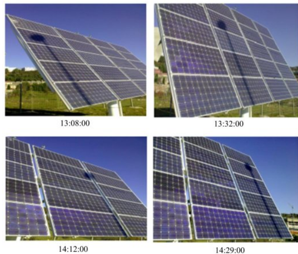
Fig. 6 Shadow caused by the lamppost
