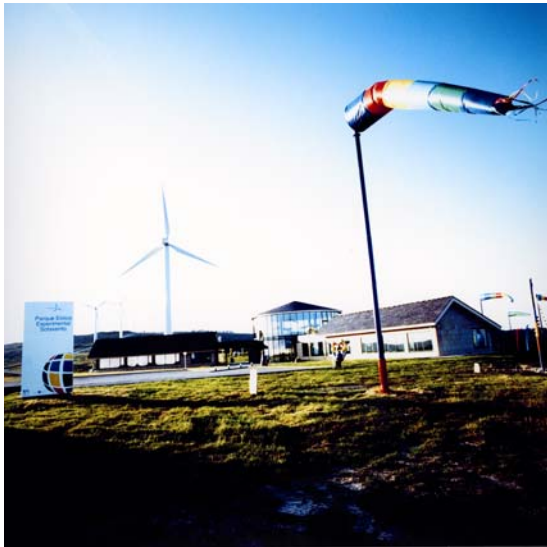
Fig. 5: Sotavento control building
